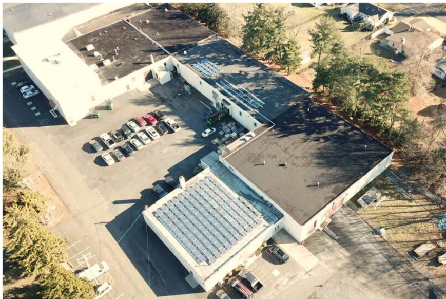
U.S Headquarters Southampton, PA
