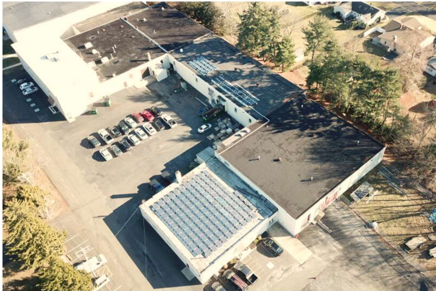
U.S Headquarters Southampton, PA
