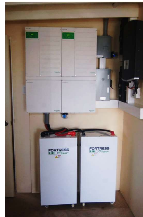
13.6 kW/30 kWh ESS
