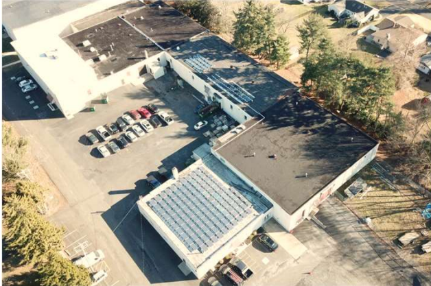
U.S Headquarters, Southampton, PA
