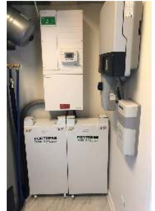
6.8 kW/30 kWh ESS
