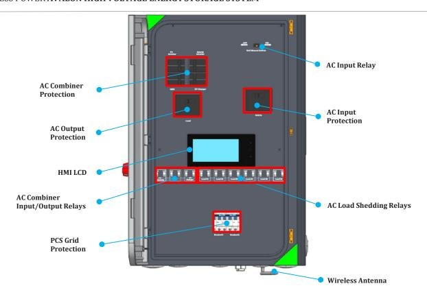
Figure 5.3 Inside Front Panel View
