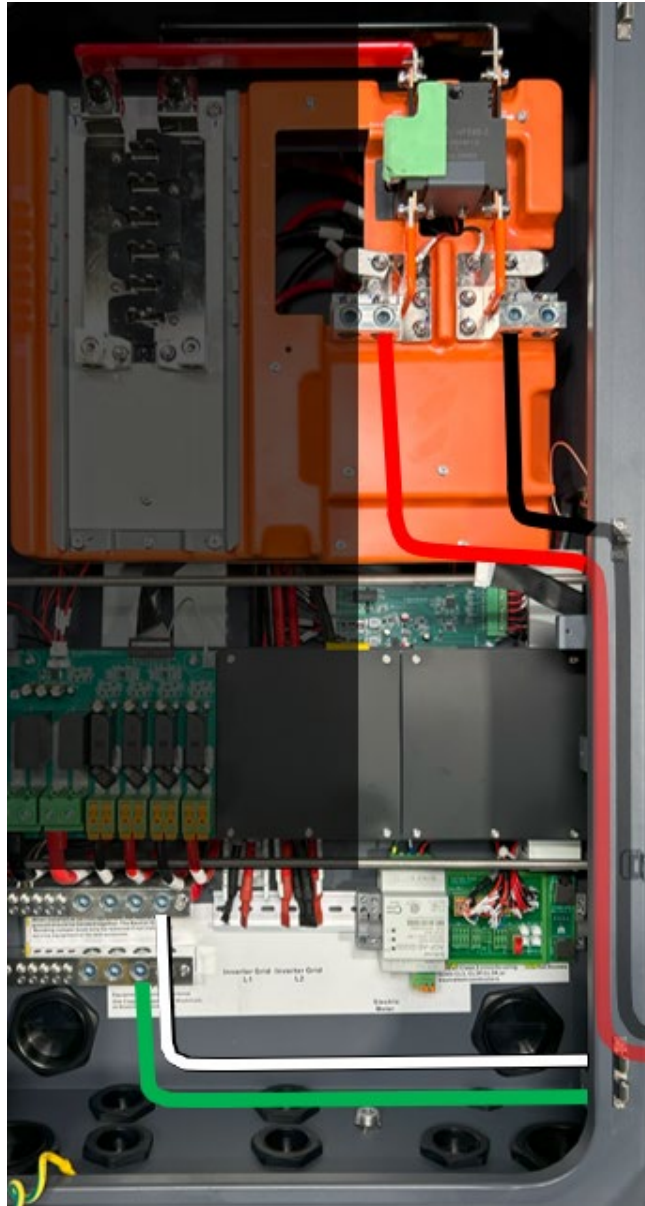
Figure 30: Inverter to Grid Interconnection
