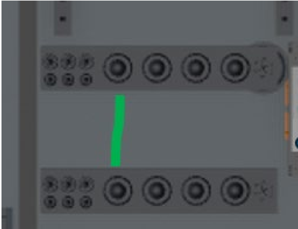
Figure 25: Neutral-Ground Bonding Location in SEP
